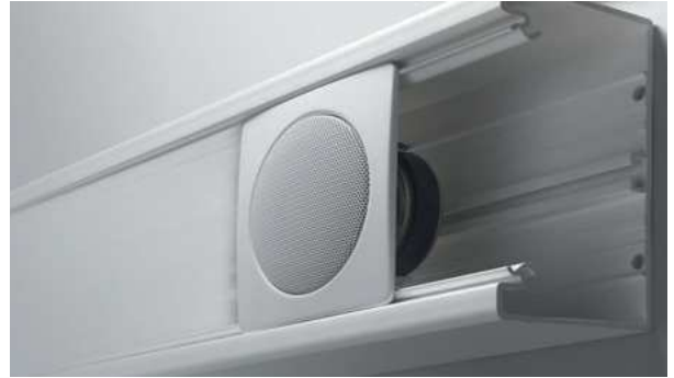
Cable channel instalation
